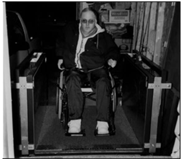
Figure 20.5. Vertical Wheelchair Platform Lift in Use.
