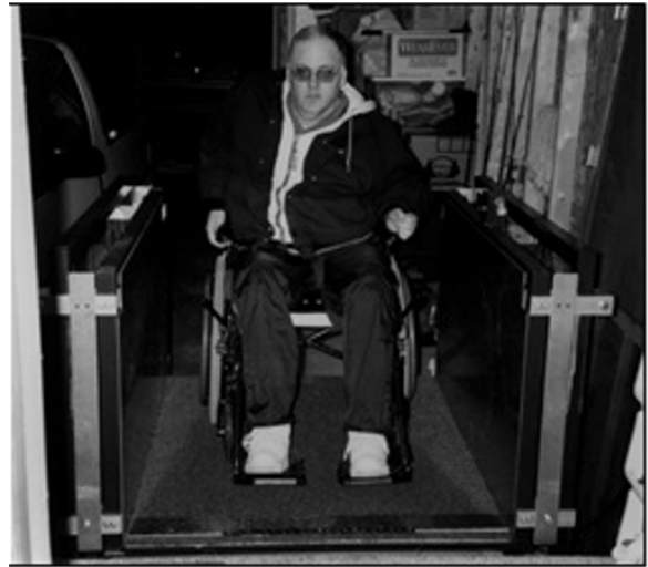
Figure 20.5. Vertical Wheelchair Platform Lift in Use.
