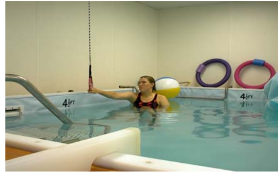
Figure 22.13. User Demonstrating the Activation of the Auxiliary Alarm.
