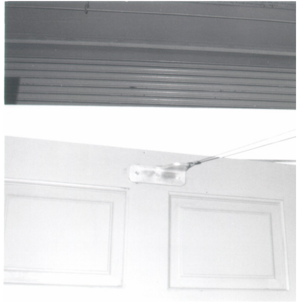
Figure 9.9. Door Plate with Motor and Spindle.
