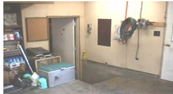
Figure 20.21. Entryway to the First Floor from the Garage Before Modification.
