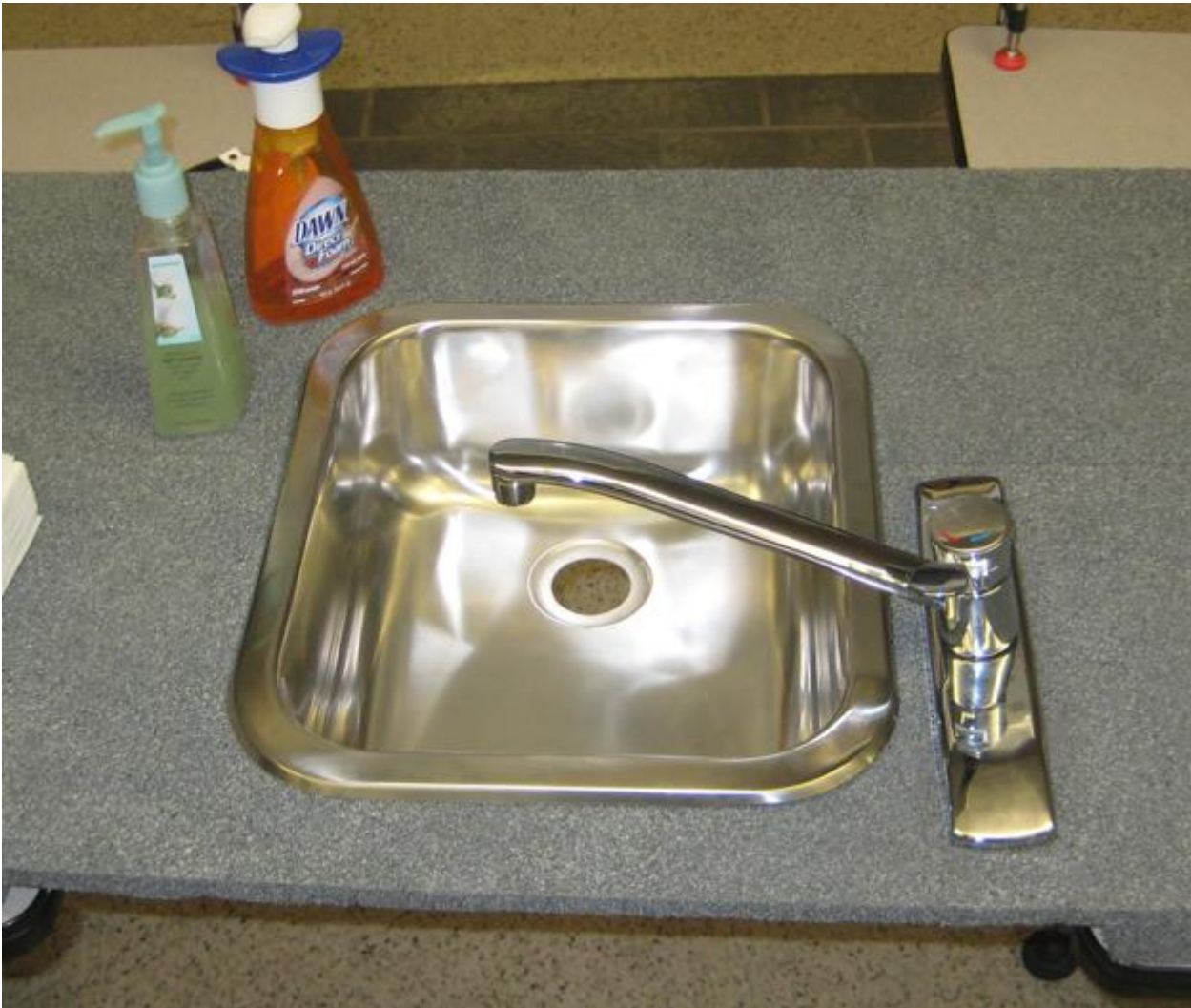
Fig. 9.10. Illustration of the installed sink configuration. Not shown is the stop that keeps the spout over the basin.
